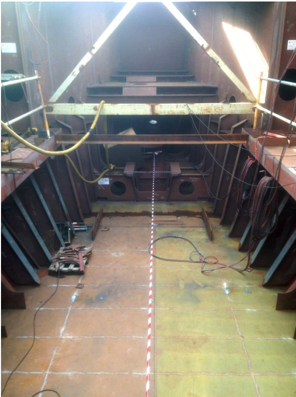
Propulsion room ready for AC motor foundations
