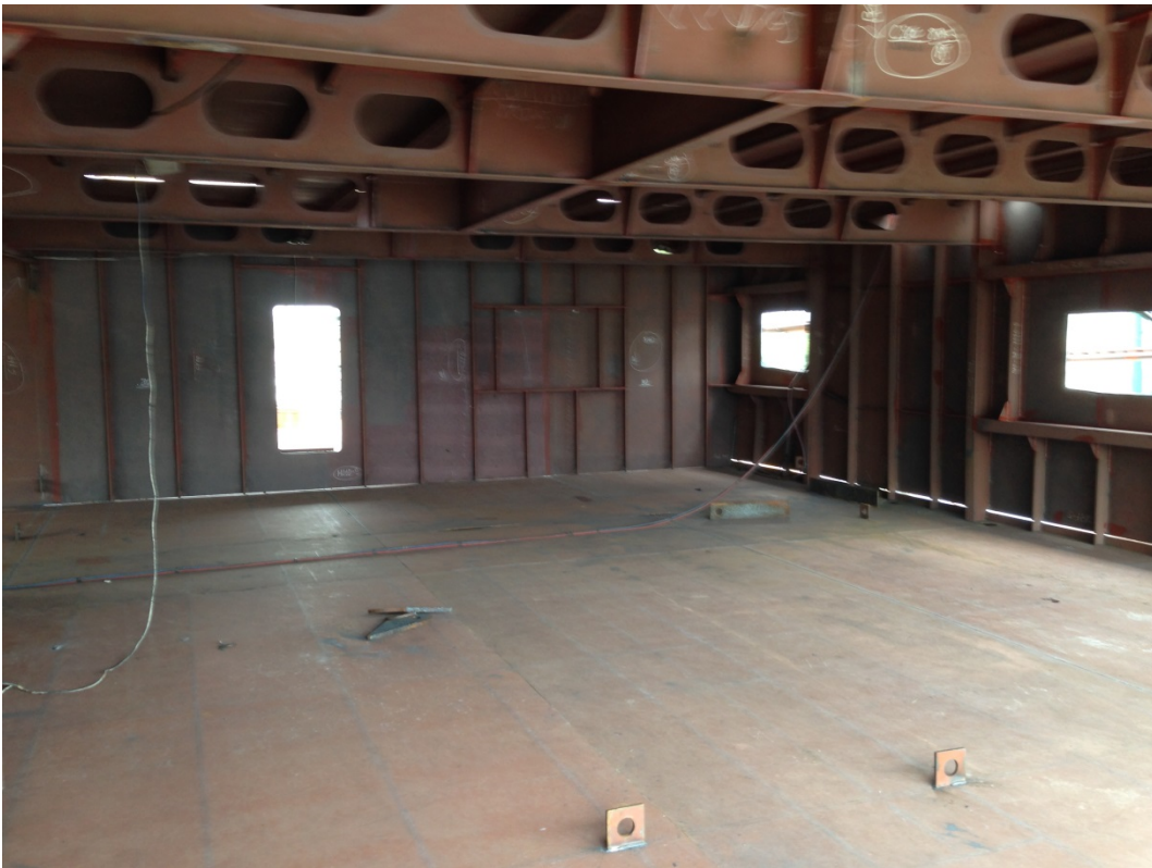
1 st dk - Messrom area w/door to galley.
